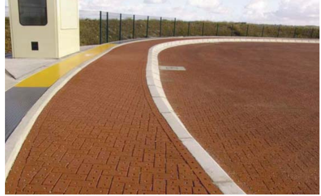
Photo 2 Permeable Clay Pavement
